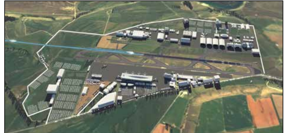
VISUALISATION OF POTENTIAL DEVELOPMENT AT WĀNAKA AIRPORT FOR THE DUAL AIRPORT SCENARIO SOURCE: ANIMATION RESEARCH AND WĀNAKA STAKEHOLDERS GROUP
