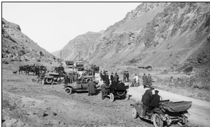
SH6 through Kawarau gorge. This is regularly upgraded by central government.
